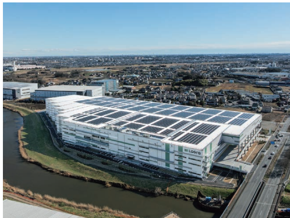
(仮称)LOGI' Q蓮田新築工事
